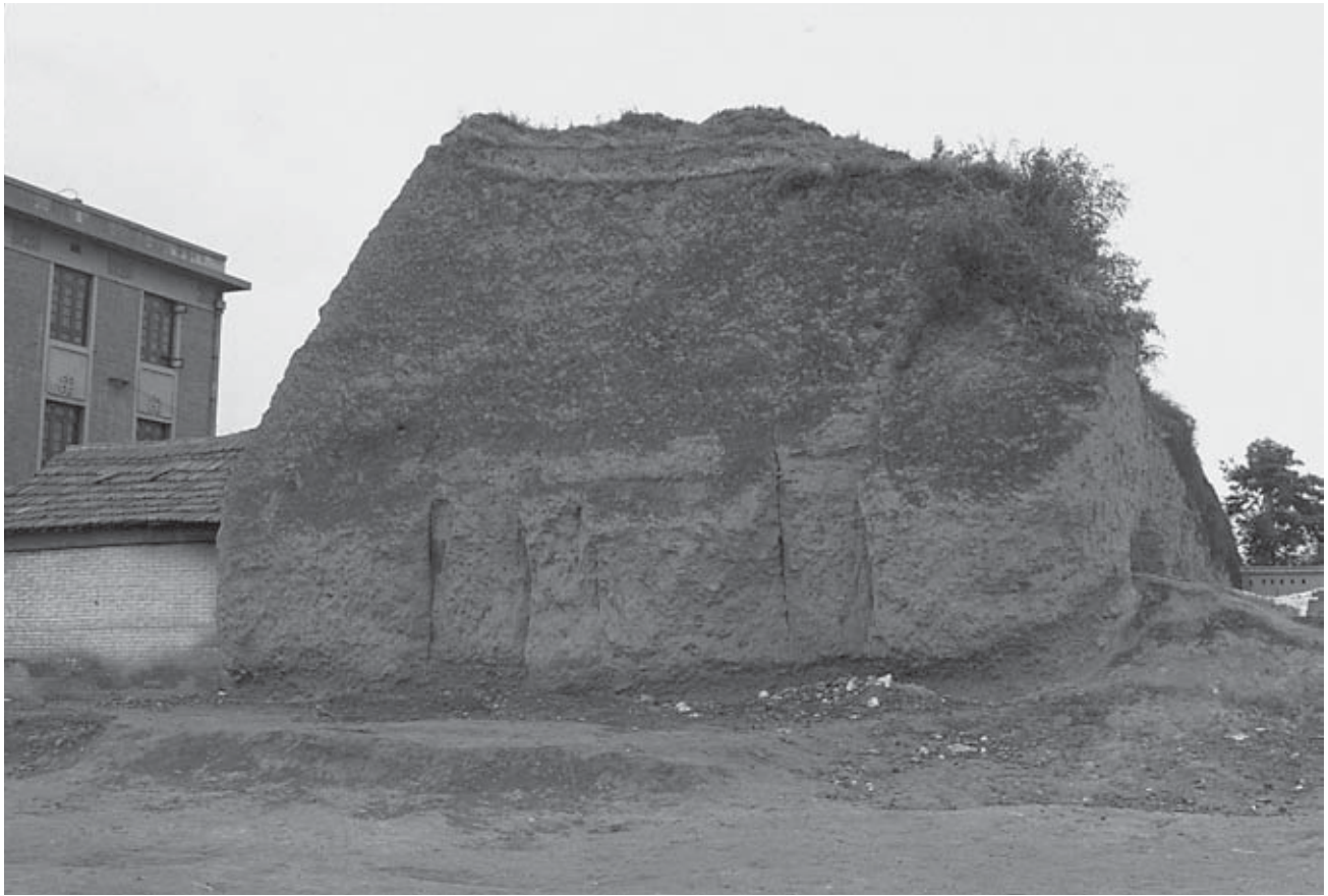
Sections of the city wall of Xi'an, originally built of rammed earth, underwent their last renovation in 1983. PHOTO BY JOAN LEBOLD COHEN.
