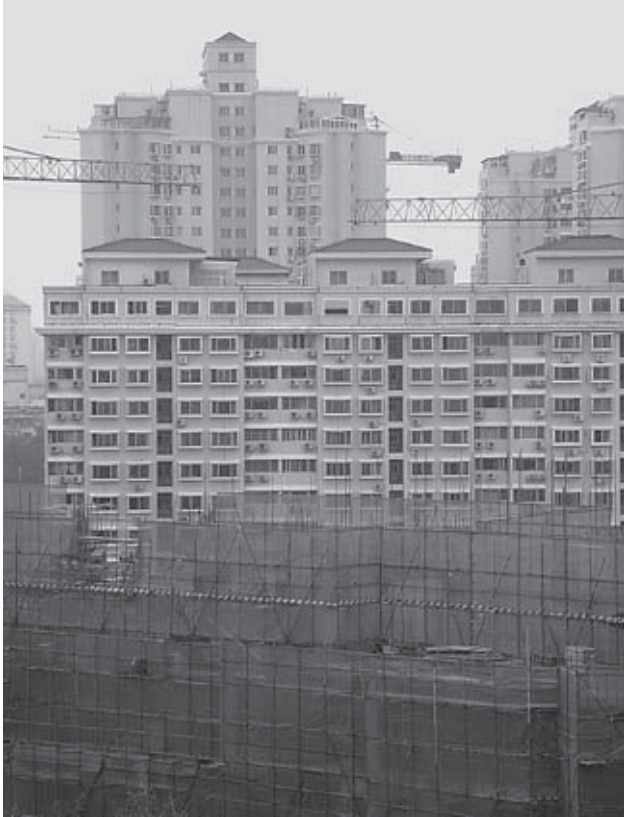
New construction spurred by urban population growth. PHOTO BY TOM CHRISTENSEN.
