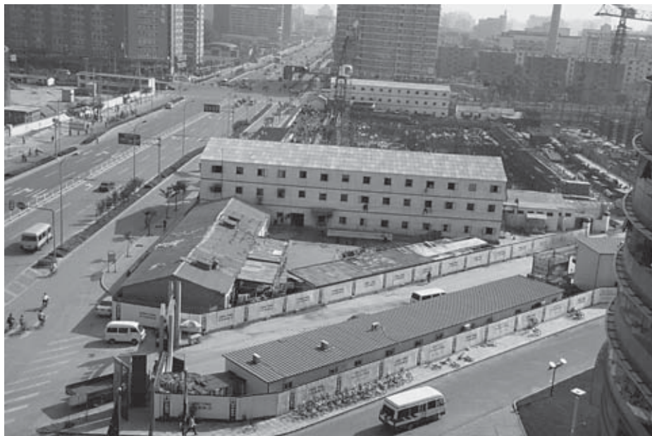
The white structure with three stories in the center of the picture is temporary housing for the migrant laborers working on the high-rise office building directly behind their quarters. Construction was finished in less than two years. PHOTO BY JOAN LEBOLD COHEN.
