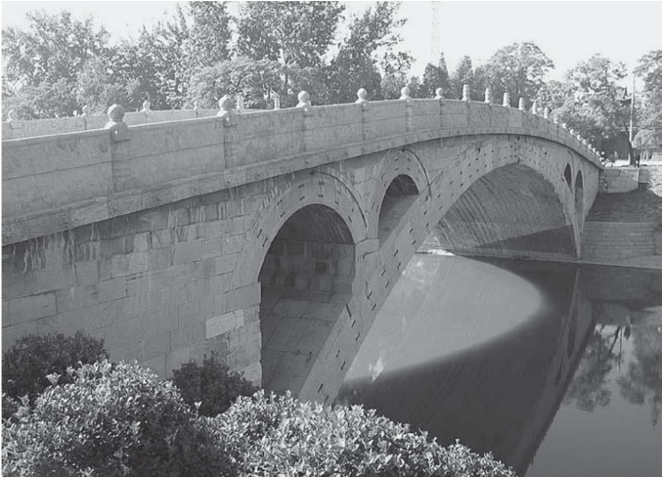
The segmented open spandrels (arches) that support the Zhaozhou Bridge, built during the Sui dynasty, were a Chinese innovation. Such engineering allowed the bridge to span a wide river and accommodate boat traffic.
