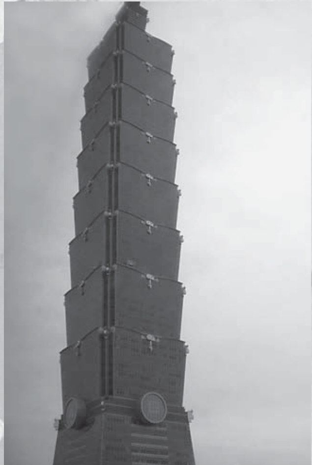
The Taipei 101 building, the tallest building in Asia. PHOTO BY JOAN LEBOLD COHEN.
