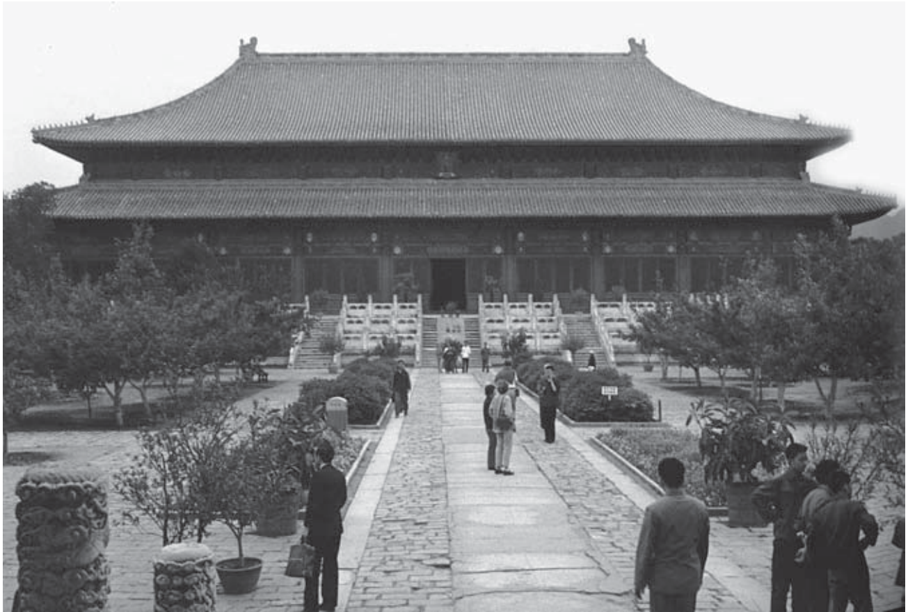
Hall of Eminent Favors, Tomb of the Yongle emperor (Zhu Di), Ming dynasty, recently renovated. This immense building is one of the largest wooden halls in Asia and, like the rest of the complex, has been extraordinarily preserved, partly because Mao Zedong paid a visit to Changling in 1954 and declared it a historical site. It was thereby spared the ravages of the Cultural Revolution. PHOTO BY JOAN LEBOLD COHEN.
