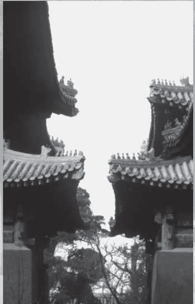
Roof eaves at the Temple of Confucius in Beijing, now the Municipal Museum. PHOTO BY JOAN LEBOLD COHEN.
